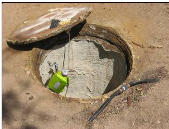
**Figure A-5.** Installed Pressure Monitor
