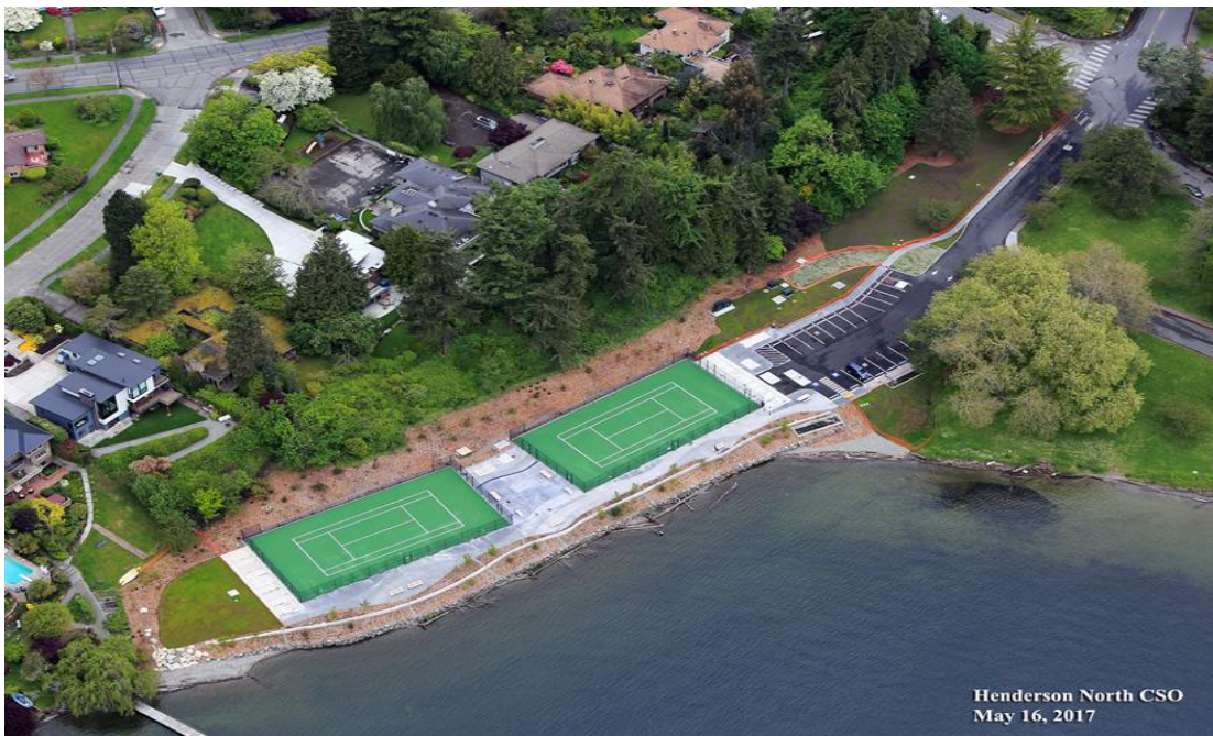
Figure 4-1. Completed North Henderson CSO Storage Facility
