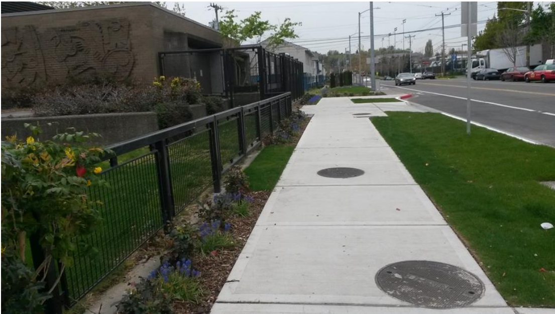
Figure 4-6. Completed 52 nd Ave S Combined Sewage Conveyance Project
