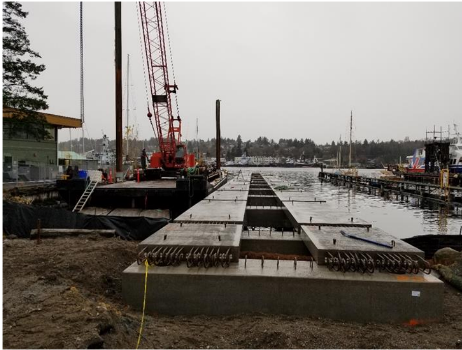
Figure 4-2. Ballard Early Work Construction – Pier Replacement
