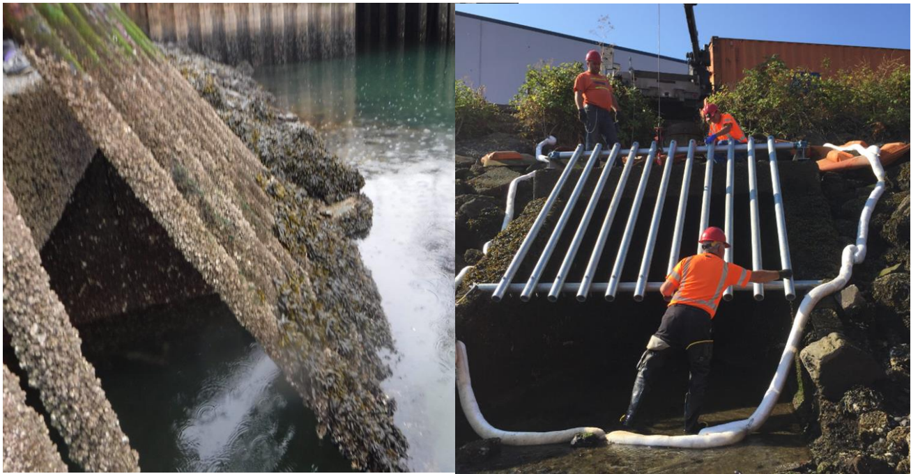
Figure 4-7. CSO Outfall 99 Trash Rack: Before and After Replacement
