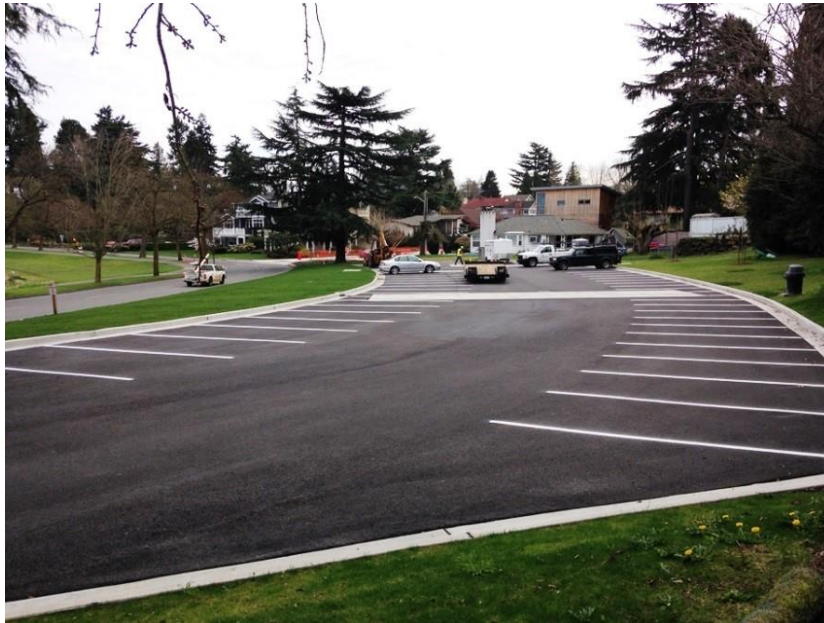
Figure 4-5. Completed Genesee CSO Storage Facility 11A
