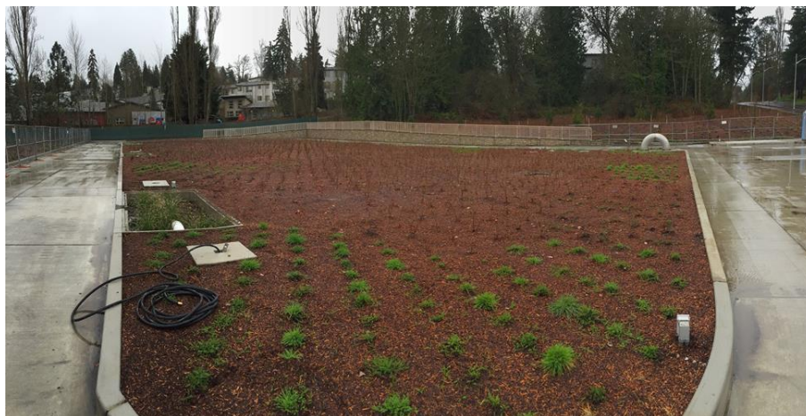
Figure 4-3. Completed Windermere CSO Storage Facility
