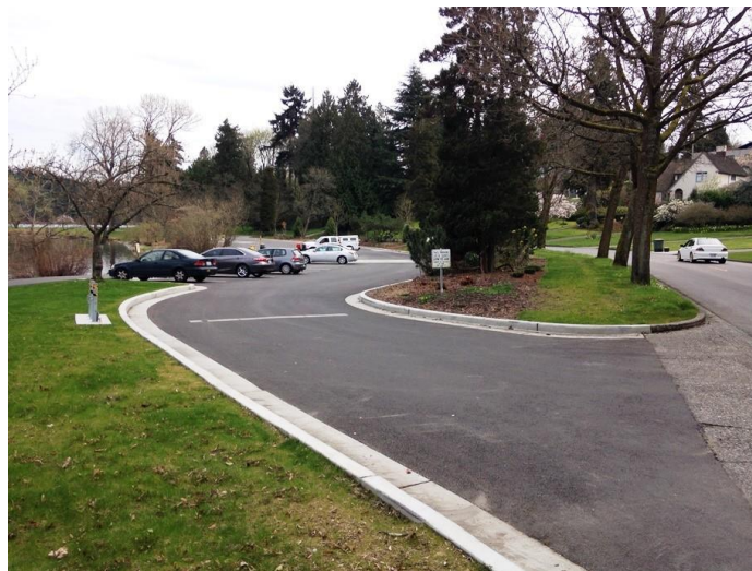
Figure 4-4. Completed Genesee CSO Storage Facility 9A
