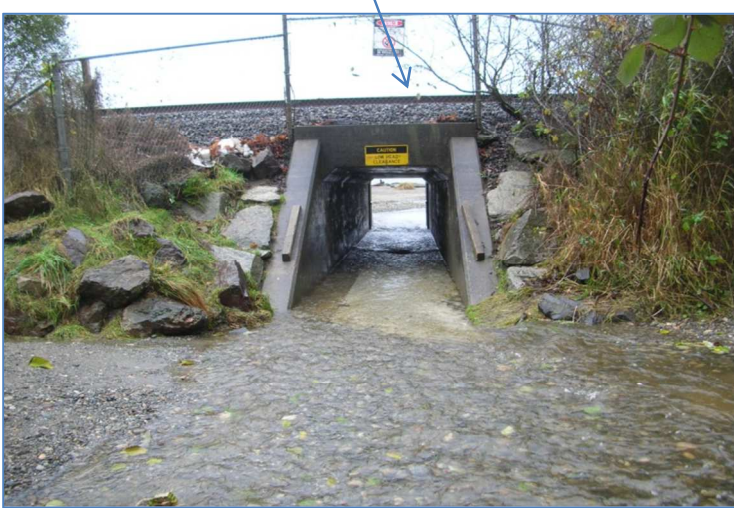
Existing Meadowdale Beach Park Culvert with BNSF tracks on top (source: www.snohomishcountywa.gov)
