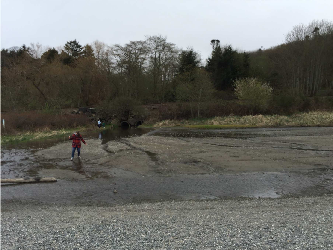
Figure 3 Existing Piper Creek Culvert at Carkeek Park
