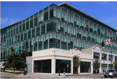
Partial preservation of the ground floor facade, with a modern addition above retains a portion of the neighborhood's history.
