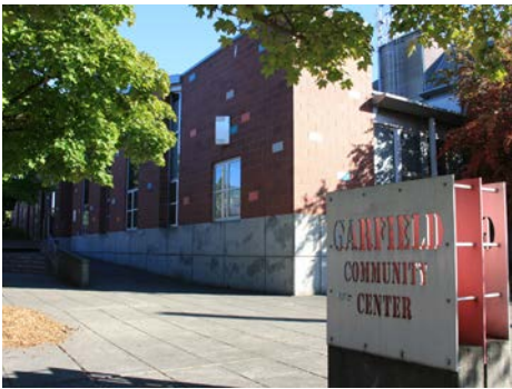
Garfield Community Center
