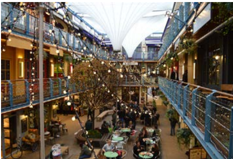
Covered gathering space that can be used throughout the year.
